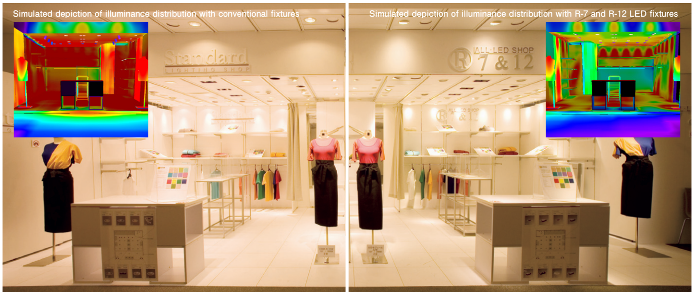
Light distribution of typical conventional fixtures
