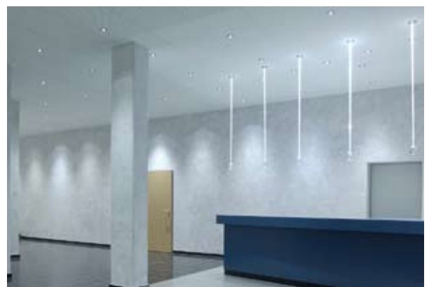
Image of the installation, Thanks to LBM
